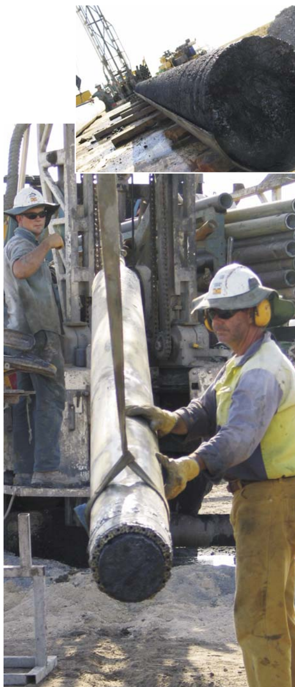
Drilling activities during the year at Lake Lindsay provided vital information allowing us to plan safe, efficient and environmentally sound development in the future.
