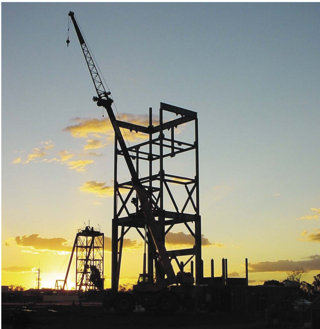
Headframes at the Grasree Project under construction.
